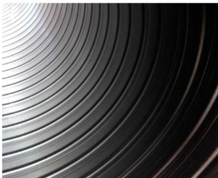
Unique seams inside Helix create the smooth surface needed for multi-directional installation
